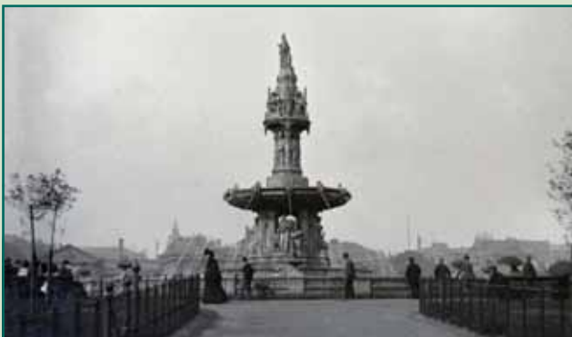
Doulton looking West
