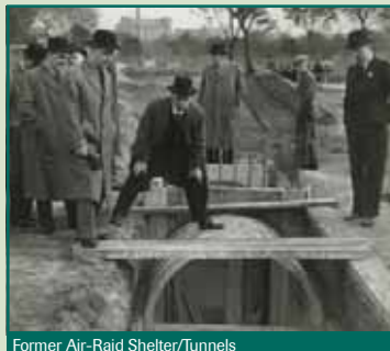
Former Air-Raid Shelter/Tunnels
