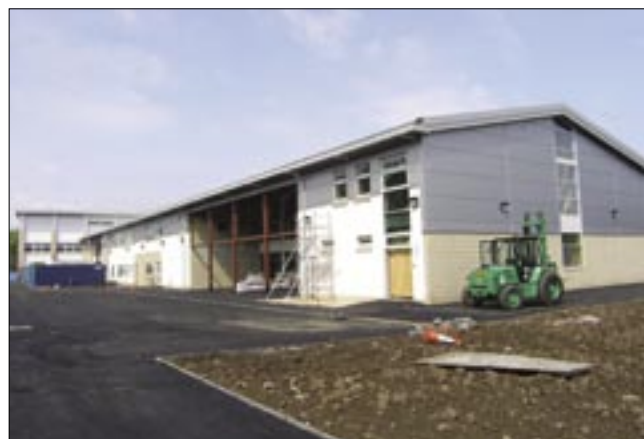
Construction of Haghill Primary School
