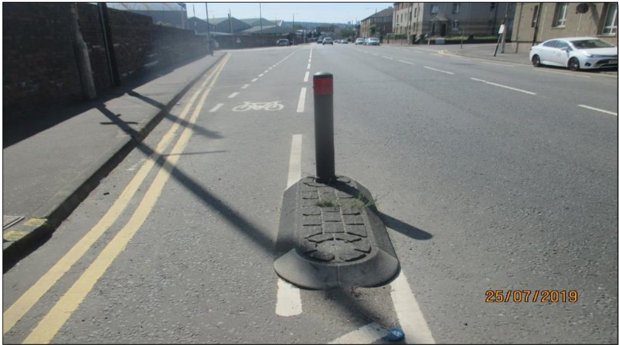
Figure 16: dividing island with missing bollard on Aikenhead Road.
