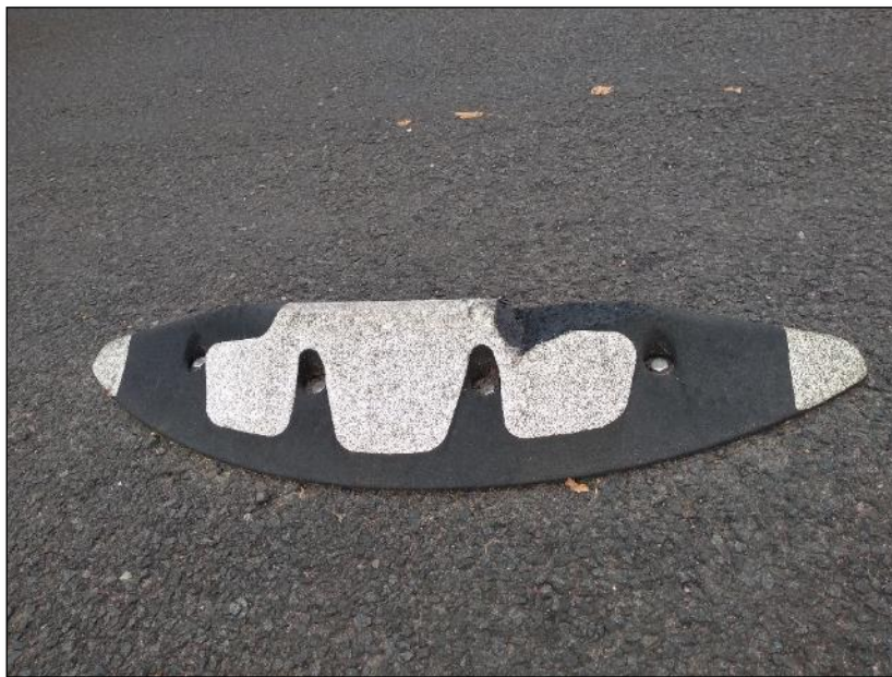
Figure 50: example of damaged Orca on Wallacewell Road.
