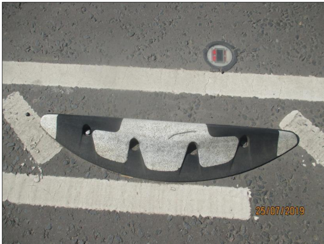
Figure 19: Orca showing signs of minor damage on Aikenhead Road.
