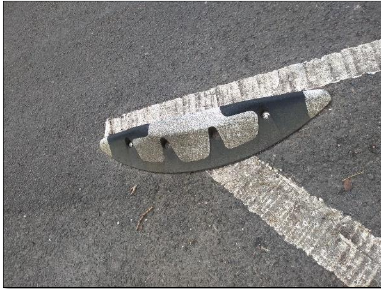
Figure 49: example of Orca's slight damage due to the unit's darkened surface as observed on Wallacewell Road.
