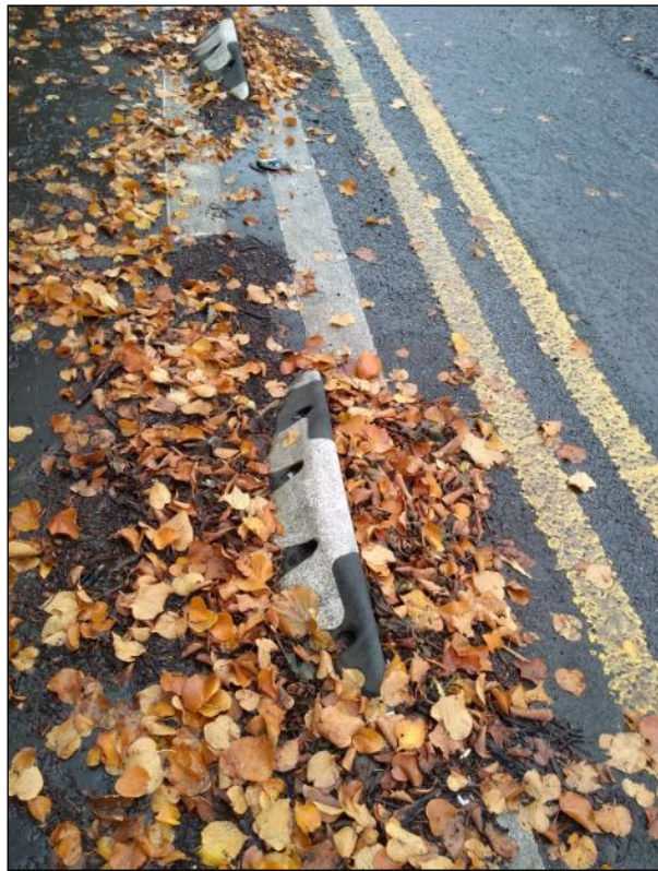
Figure 29: example of weepers blocked by debris/slit along the routes to Knightswood Park.
