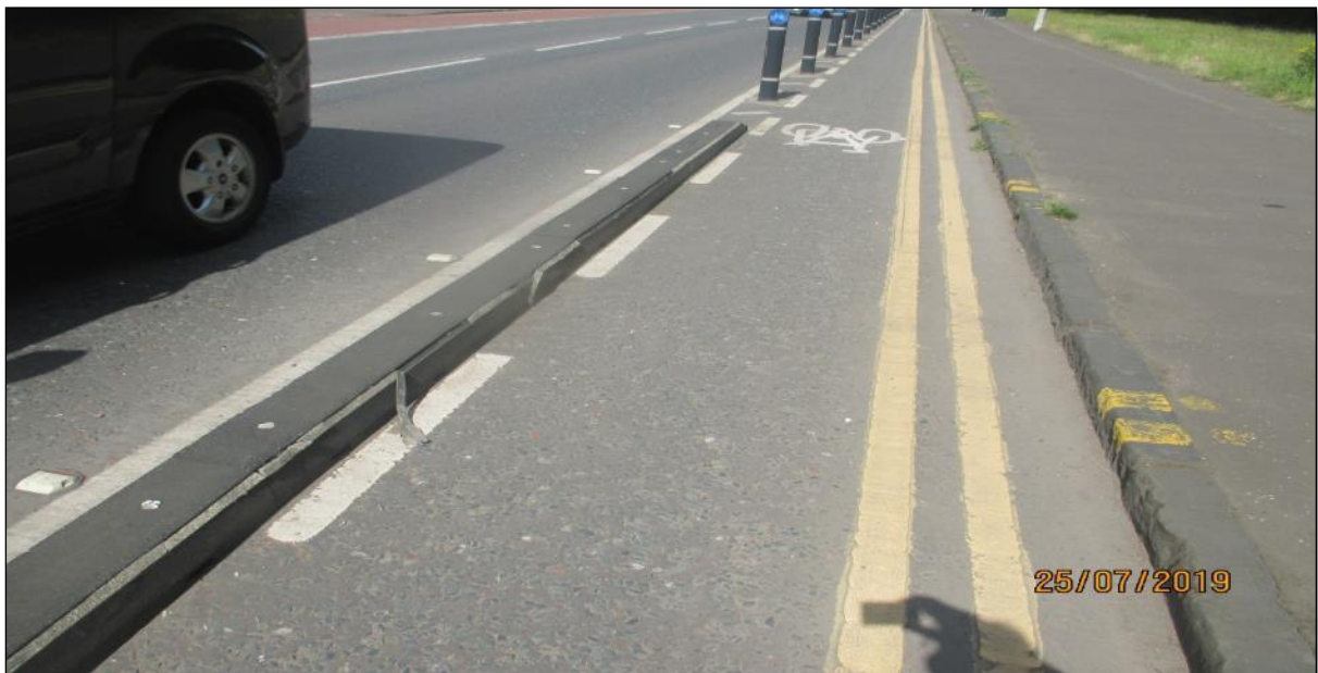
Figure 22: example of Cycle Lane Defenders showing slight damage due to reflective strip peeling off.
