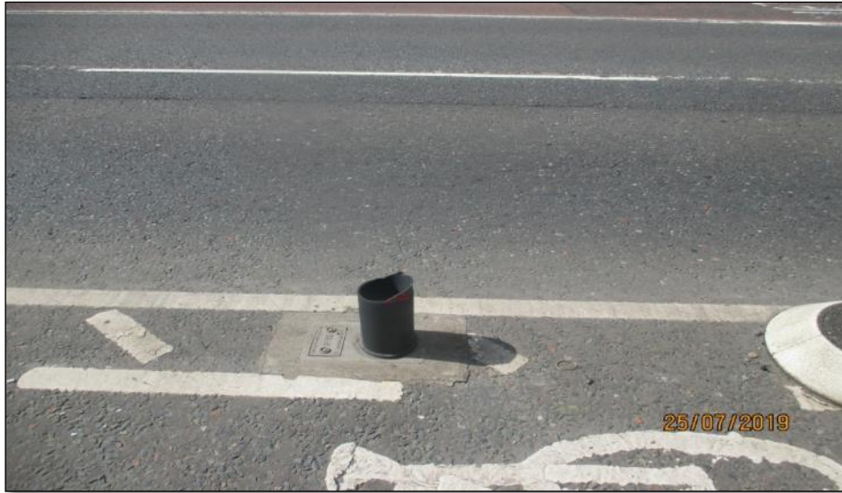
Figure 8: damaged bollard on Aikenhead Road.
