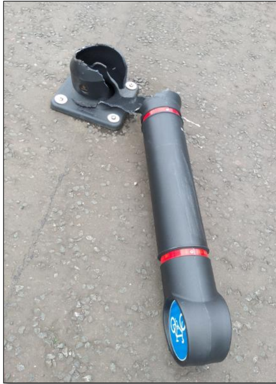
Figure 44: example of damaged bollard on the River Clyde South Bank Route.
