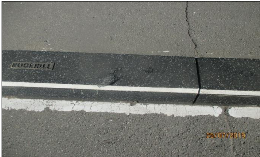
Figure 54: example of damaged Defender on Berkeley Street.
