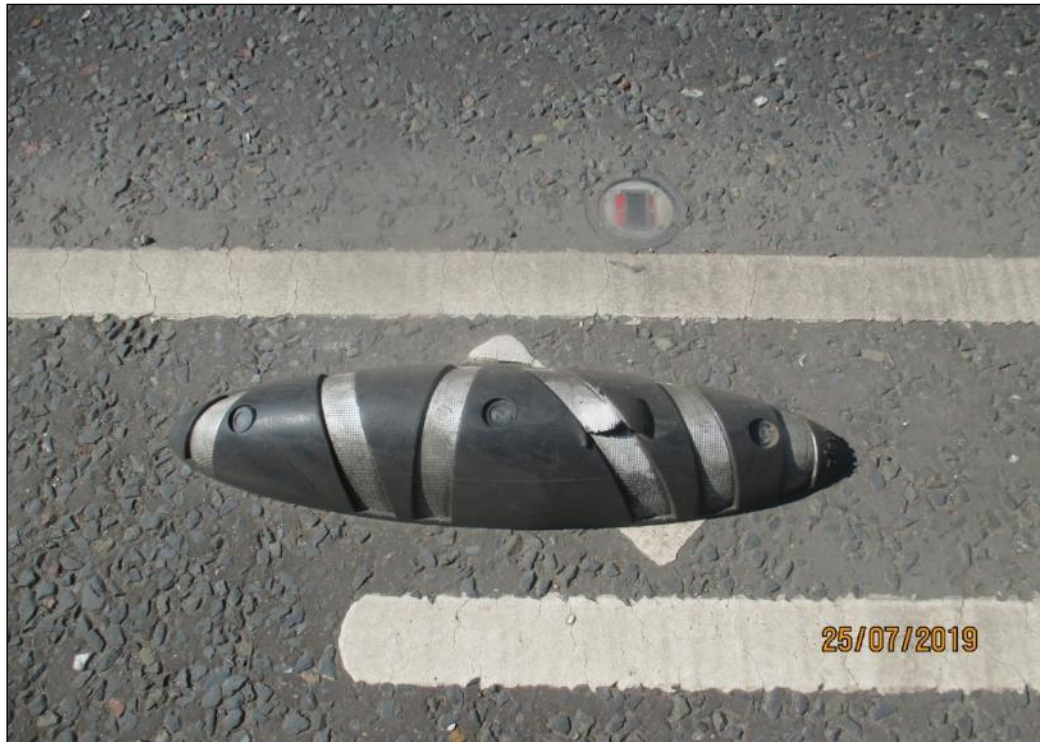
Figure 13: example of damaged Armadillo on Aikenhead Road.
