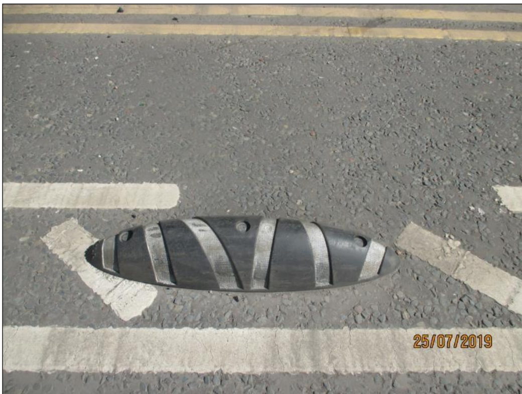
Figure 14: Armadillo defender showing signs of discolouration within reflective area on Aikenhead Road.
