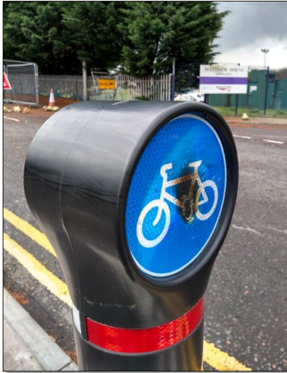
Figure 35: damaged bollard presenting signs of vandalism along the routes to Knightswood Park - Dyke Road.
