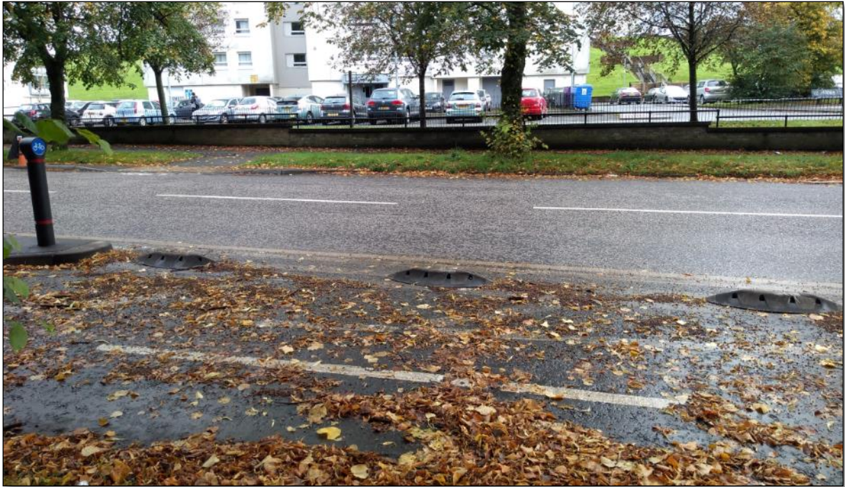
Figure 32: example of Orcas showing major damage due to extremely darkened surface along the routes to Knightswood Park.
