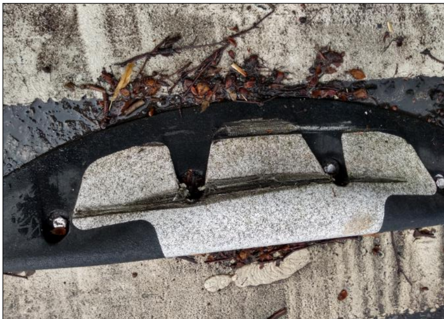
Figure 31: example of Orcas showing major damage to the top surface along the routes to Knightwood Park.
