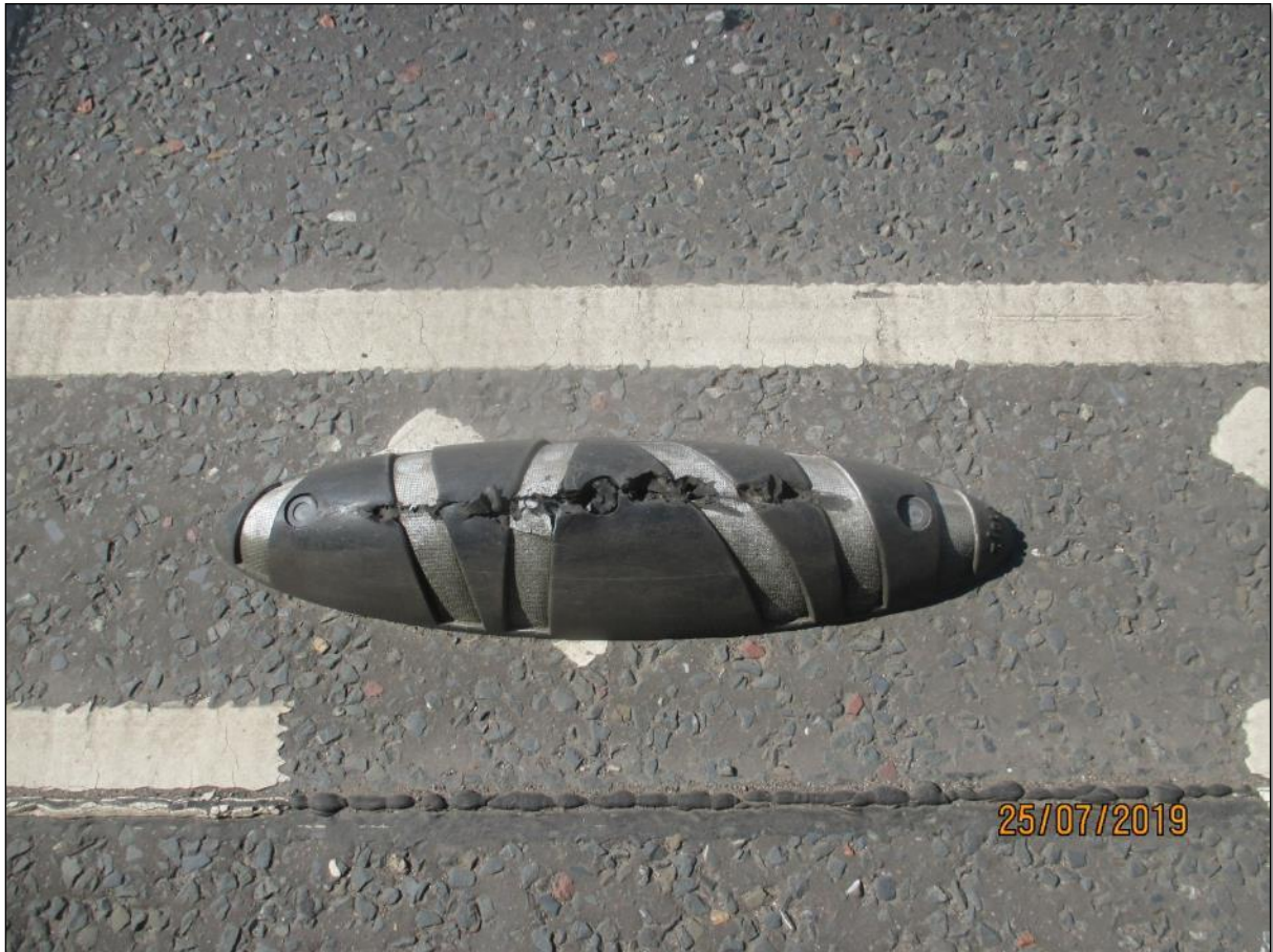
Figure 12: example of damaged Armadillo on Aikenhead Road.
