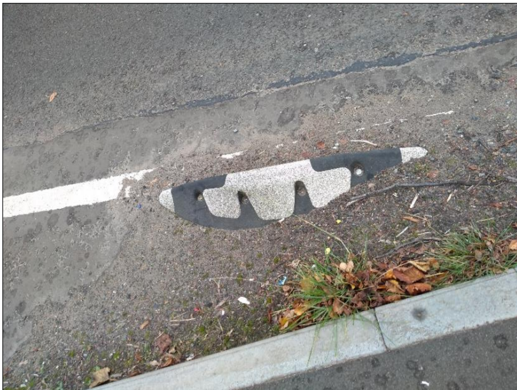
Figure 48: example of Orca's weepers blocked by debris/slit on Wallacewell Road.
