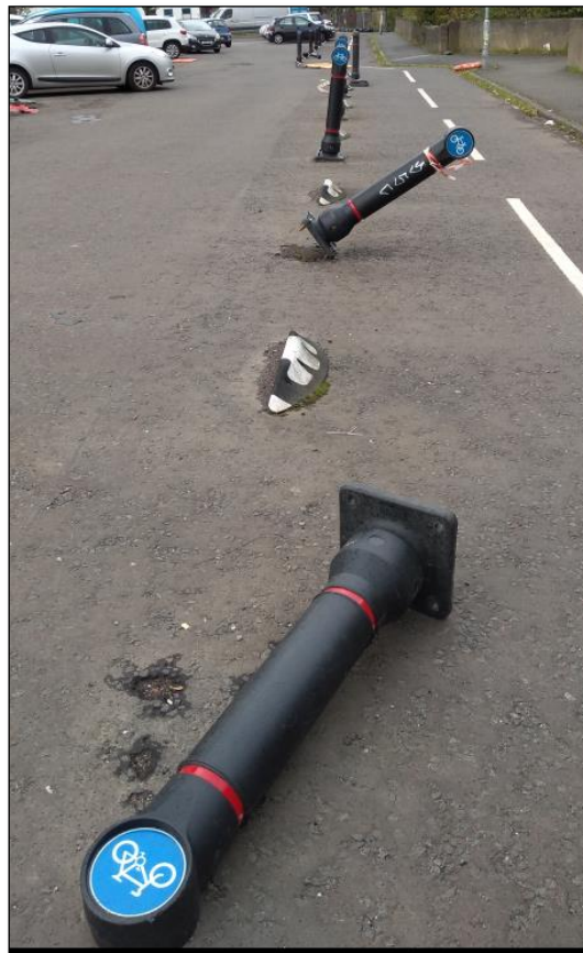
Figure 45: example of a displaced bollard and a unit with loose/missing bolts on the River Clyde South Bank Route.
