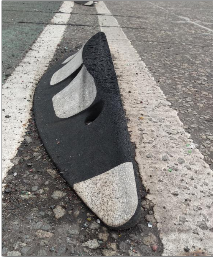
Figure 26: example of major damage to Orca on Glasgow Bridge.
