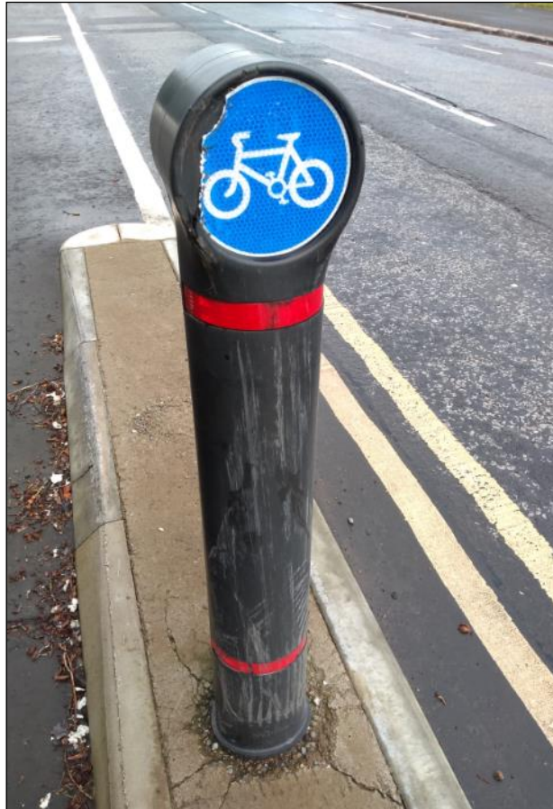
Figure 34: damaged bollard along the routes to Knightswood Park - Dyke Road.
