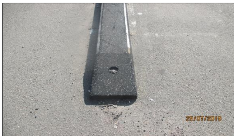
Figure 55: cycle lane Defender on Berkeley Street showing signs of minor damage.
