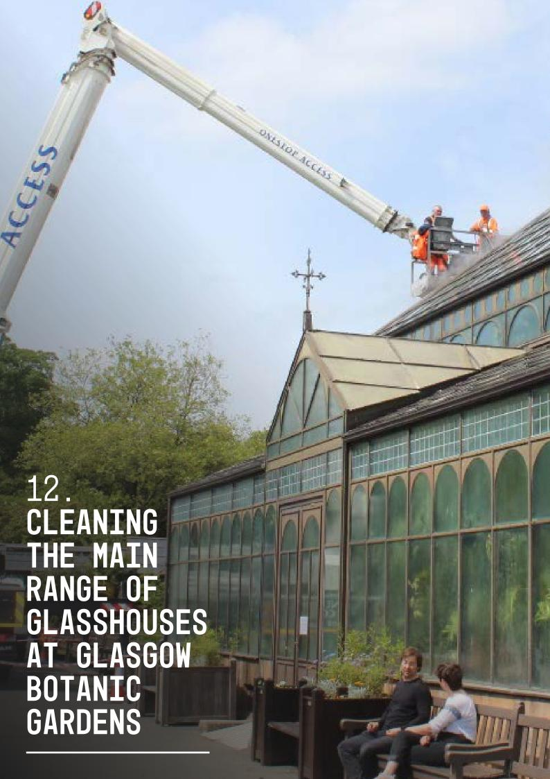
One of the tasks carried out at Glasgow Botanic Gardens is the cleaning of glass at high level both in the Kibble Palace and the Main Range of Glasshouses. This task normally involves the hire of high-level access equipment over a long period of time with down time in cleaning often used to gain access to high hedges for seasonal maintenance.
