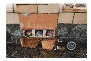
Terracotta is a fragile material, prone to frost damage. The two years of Covid have not been kind to the fountain, so an inspection in May 2022 revealed that the fountain required a significant amount of repairs by skilled artisans.
