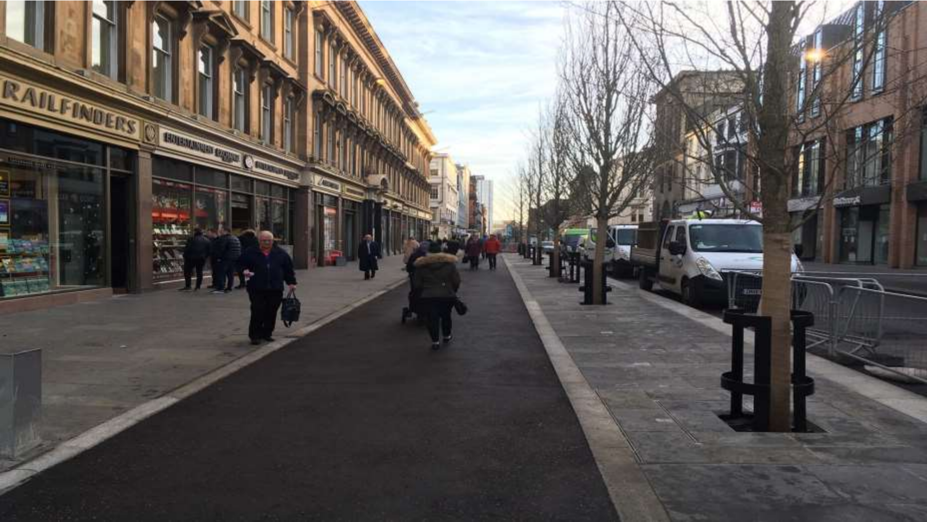
Appendix 2: Sauchiehall Street West: Avenue mid-construction (January 2019)
