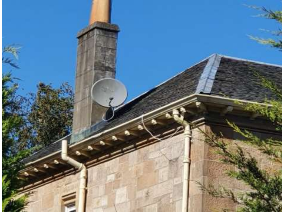
Plate 7. Roof at front of building (southern end), gap under ridge end etc.
