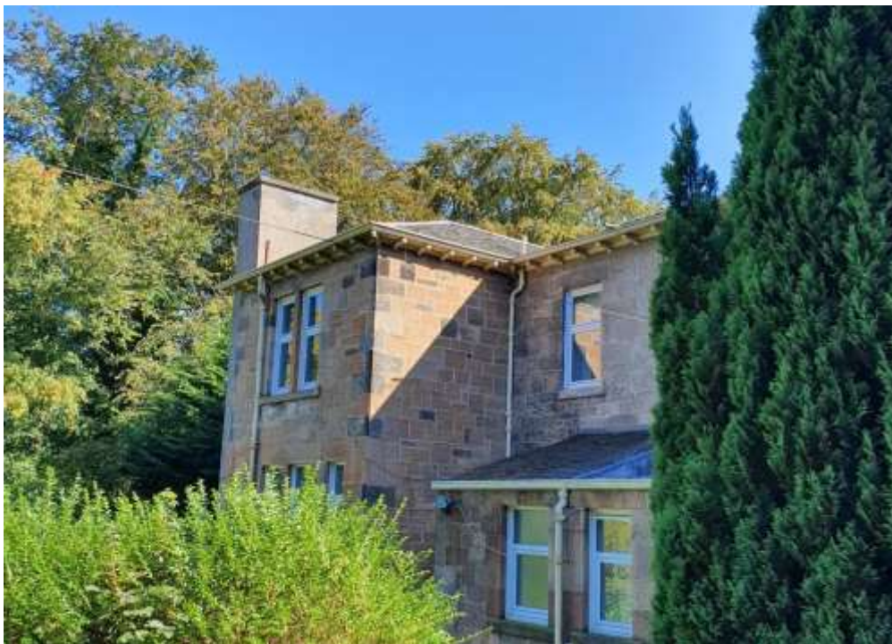
Plate 8. Rear of building (façade facing northwest)
