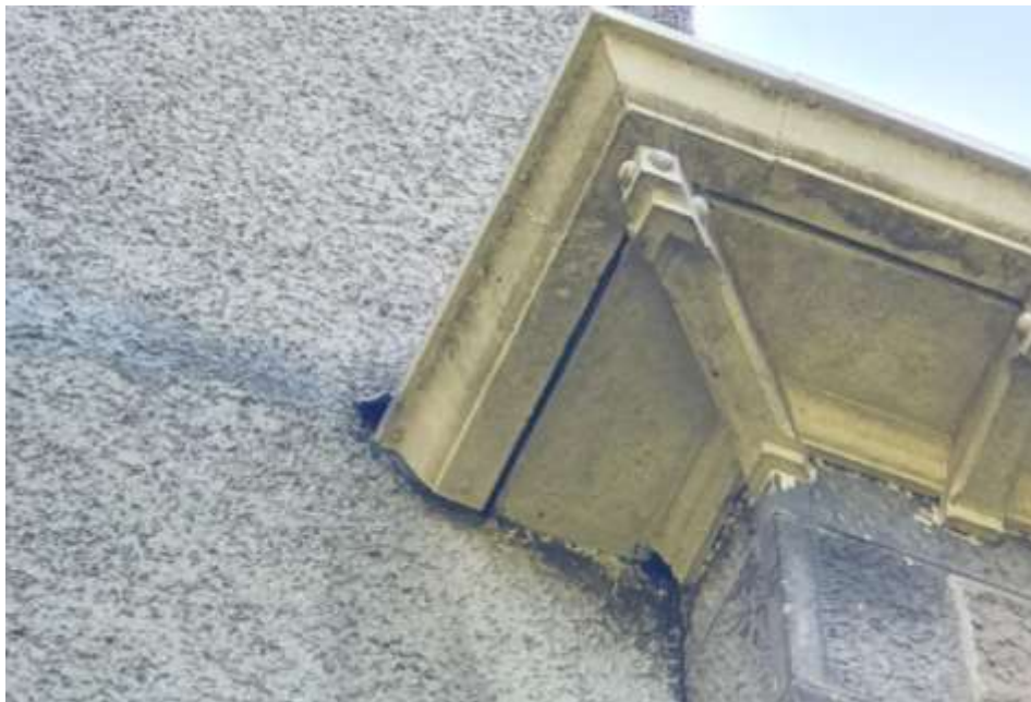
Plate 4. Rear of building (northern end by chimney) gaps under flashing and crevice to rear of soffit
