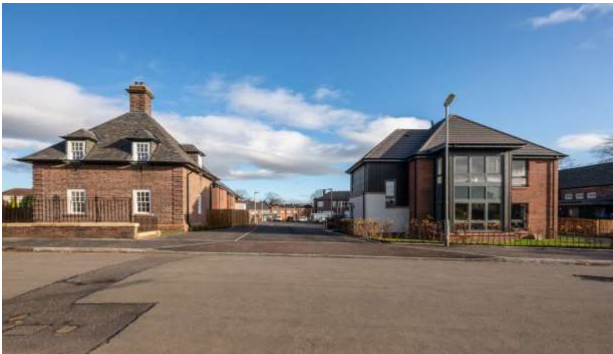
Buckley Street – Loretto Housing Association
