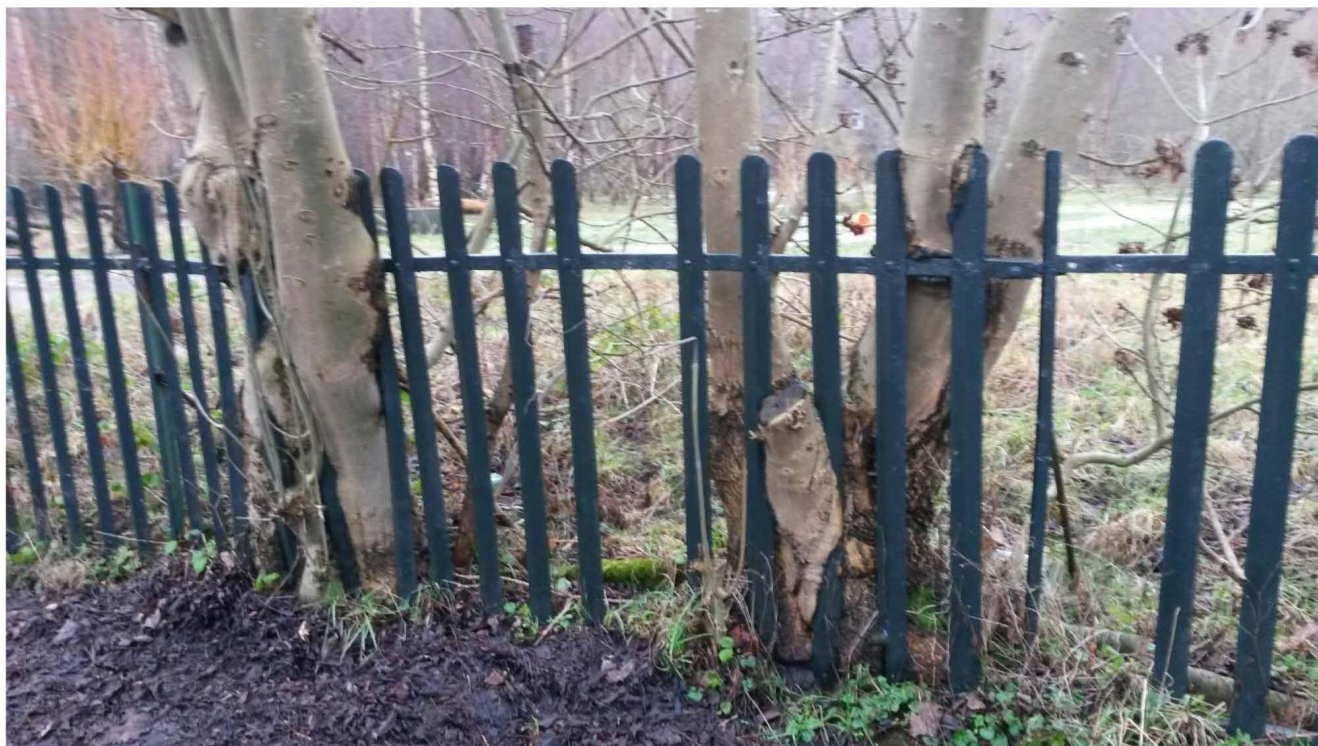
Photograph 8: Trees damaging the boundary fence on Kelbourne Street
